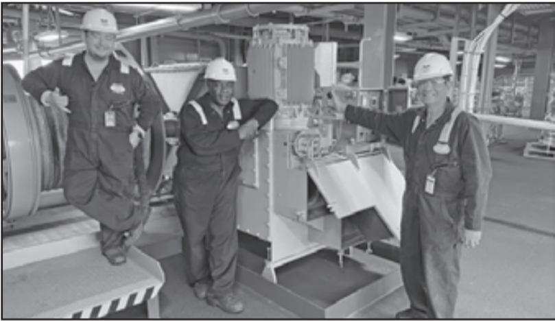
ABOARD USNS HARVEY MILK – Many thanks to AMO member Capt. Doug Voss for this snapshot from the new vessel's sea trials. The union-built ship (General Dynamics NASSCO) will be crewed by SIU CIVMARS for the Military Sealift Command, but the SIU and Seafarers-affiliated AMO provided manpower for the sea trials. "The SIU crew did an excellent job," Voss noted. Pictured from left are AB James Zaro, AB Edward Mills and Recertified Bosun Renato Govico.
