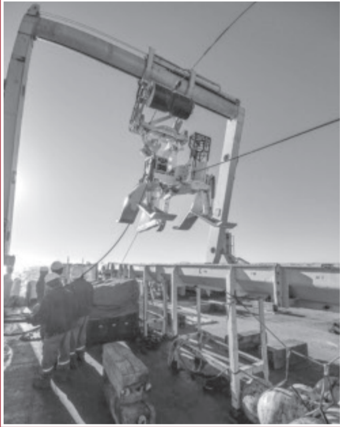
Crewmembers aboard the CS Decisive (photo above) prepare to bury cable using a device called a Plough. In addition to burying the cable two meters under the ocean floor, the mechanism also lays the cable. In the photo at immediate right, a vessel hauls shore end cable to the beach where ultimately it will be connected to a shore side station. Thanks to Recertified Bosun Victor Nunez for providing these photos.
