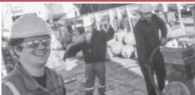
AB/Third Mate Tyler Brenton (left), AB/SJ Arsenio Brecio (center) and AB Paul Nelson apply floats to the umbilical cord of the Plough prior to launching it to begin the cable burial.
