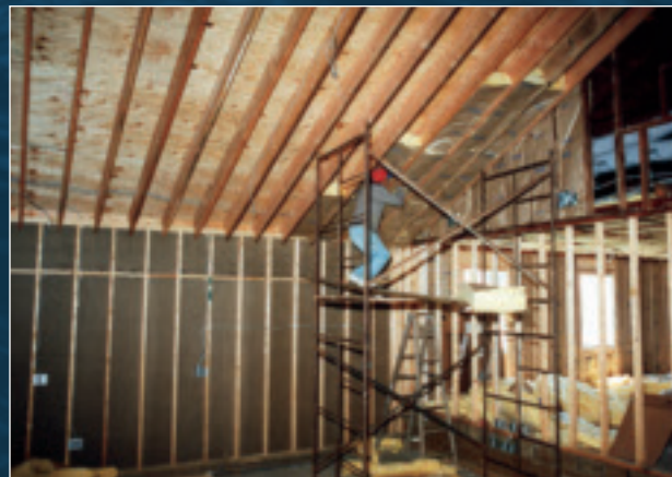
1992 ushered in the construction of a revamped Steward Department culinary lab. Here, workers install insulation in the new building.
