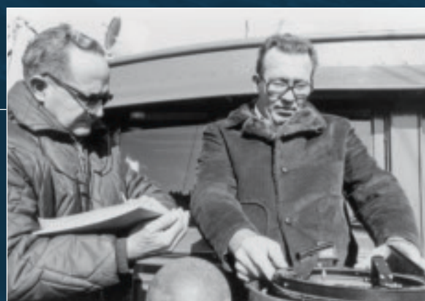
Boatmen Leonard Downs and Sam Rowe taking bearings with a gyro-repeater, 1976.
